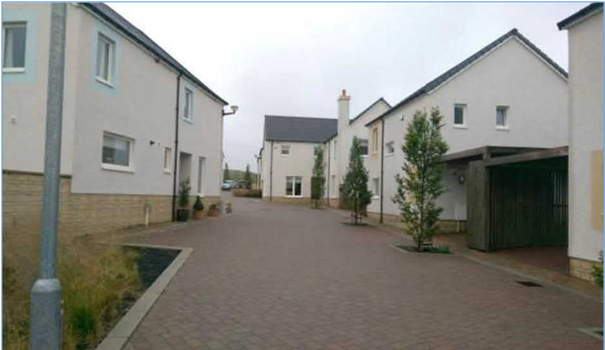
Figure 6: Close Proximity of Buildings
